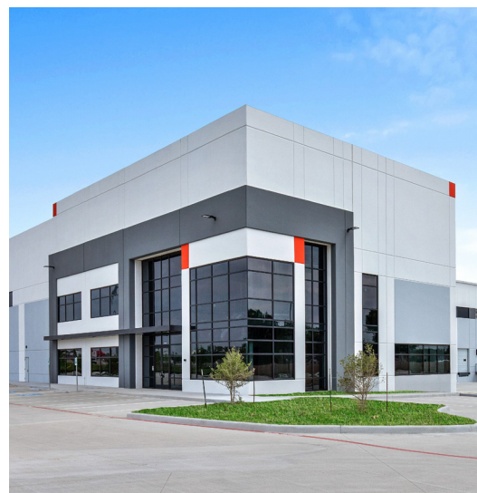
225 Logistics Center, Houston, TX
